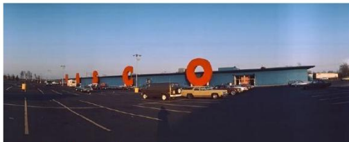
Venturi and Rauch, Basco Building, Philadelphia, 1979
